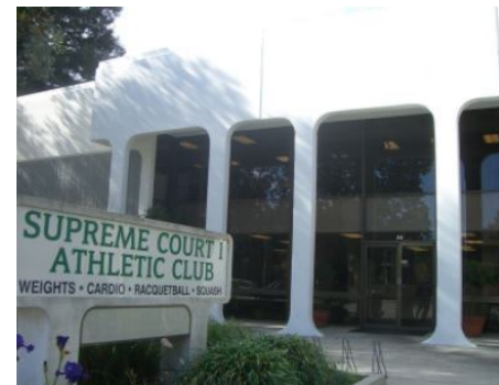
Example of a tilt-up structure remodeled to incorporate a more prominent entry with an attractive use of materials, design, and public art. Image Credit: Hillhouse Construction Company
