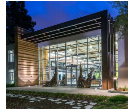
Example of a tilt-up structure remodeled to incorporate a more prominent entry with an attractive use of materials, design, and public art. Image Credit: Hillhouse Construction Company
